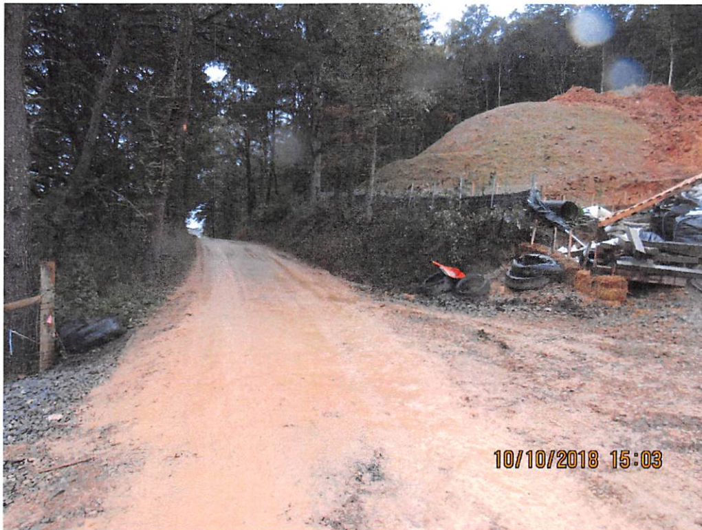
Photo 4: Painter's Run Road station 10270 at access road crossing.
