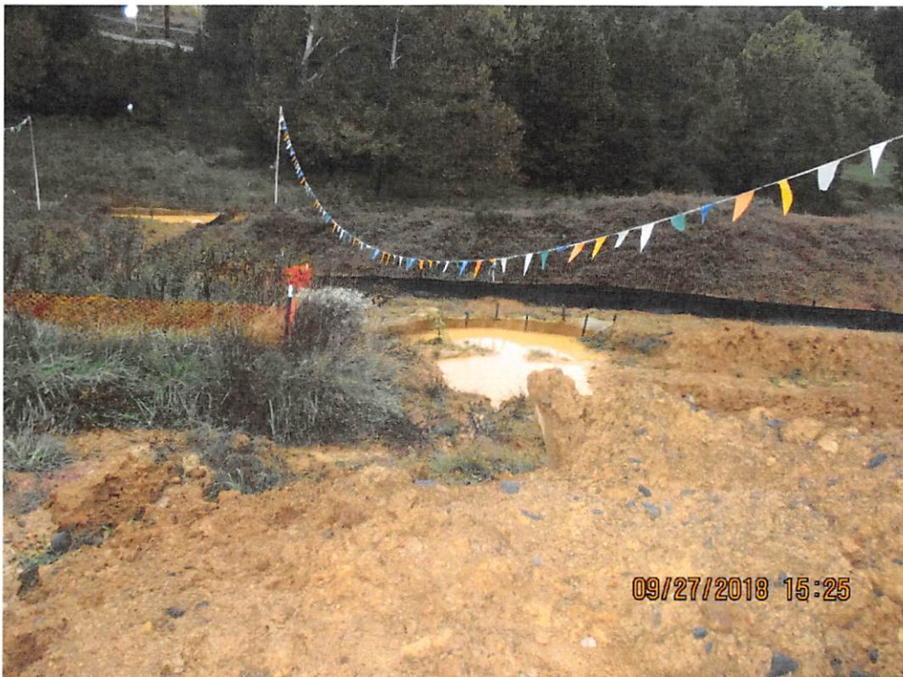
Overview of slope leading towards Stream (S-A60) near station number 9639+00.
