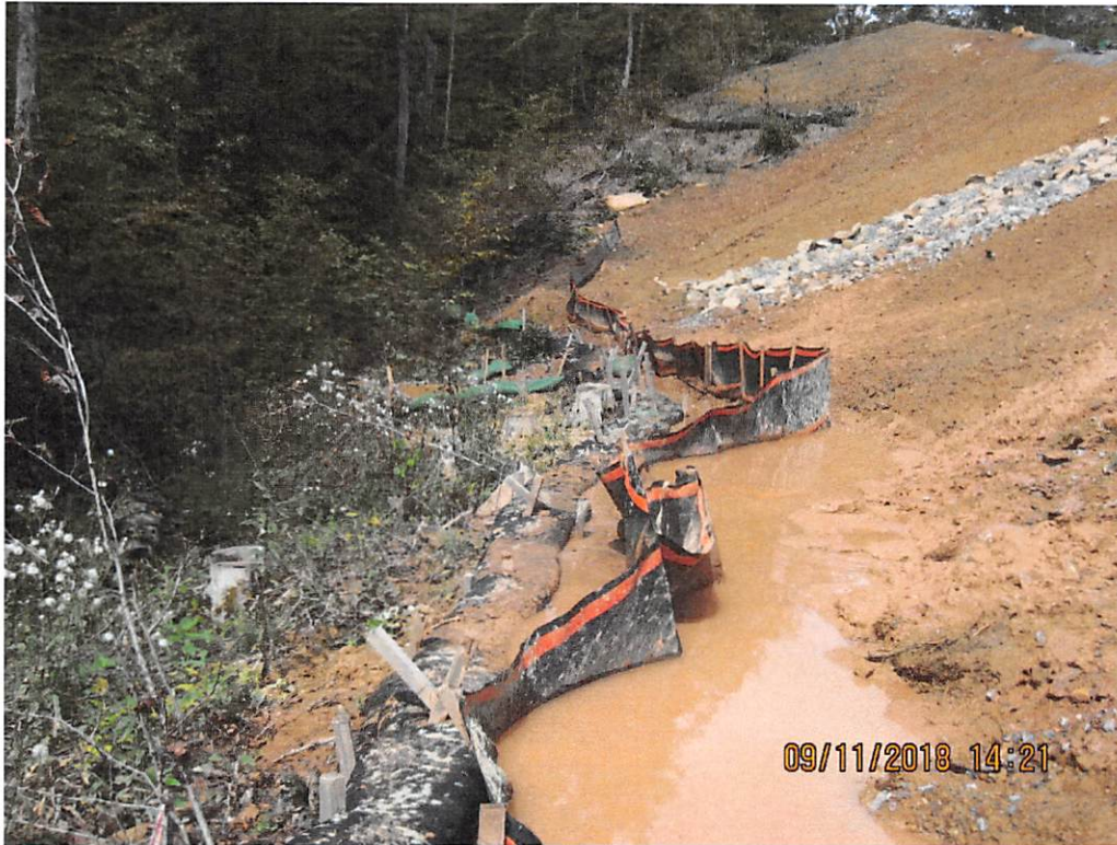
Photo 7: Station 900 (approximately) -Flow along silt fence from culvert outlet downslope to sump.
