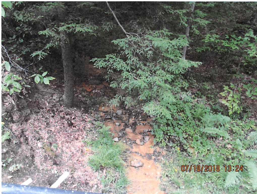
Photo 8: Sediment deposits in UNT of Harmony Creek below 1 st water bar failure
