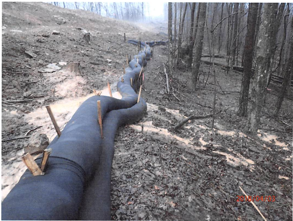
Second site of sediment laden water leaving site at Bradshaw Compressor Station.
