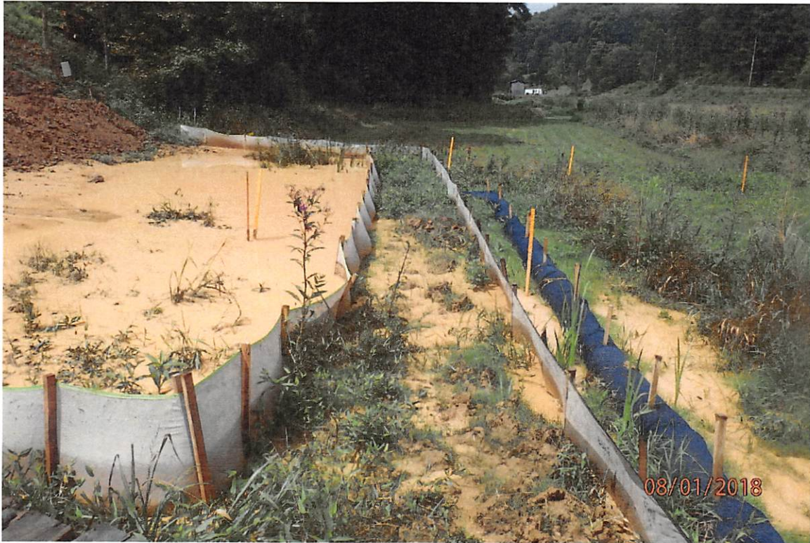
Perimeter controls adjacent to Big Elk Creek that are overwhelmed due to improperly installed water bars.
