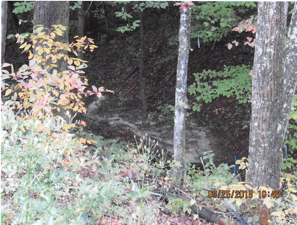
Photo 3: Conditions not allowable in UNT of Little Kanawha River down gradient of photo 2.
