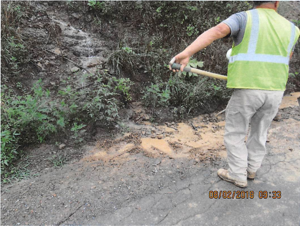
Water bar discharge mixing with sediment in road side ditch with crew performing maintenance.
