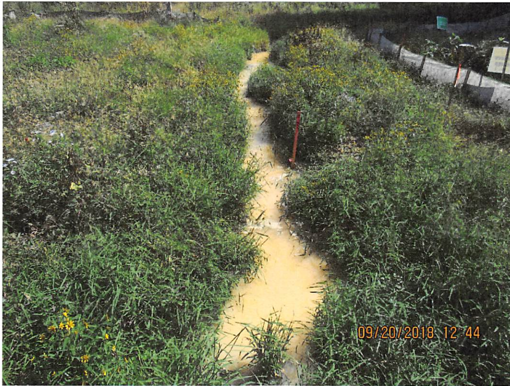
Photo 1: Plume in UNT of Painters Run from control failure off access road 231.01 near station 10270+49.
