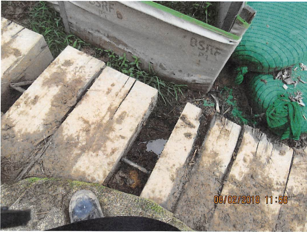
Sediment laden water traced under bridge matting.
