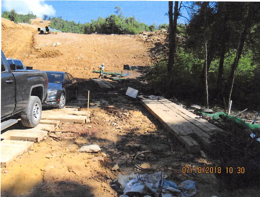
Photo 5: Upslope view of station 6898+59.
