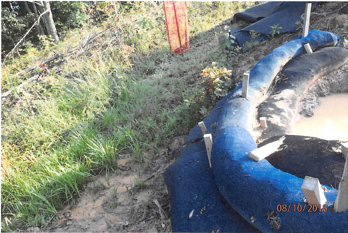
Water bar terminus that discharges onto MVP-DO-049 access road.
