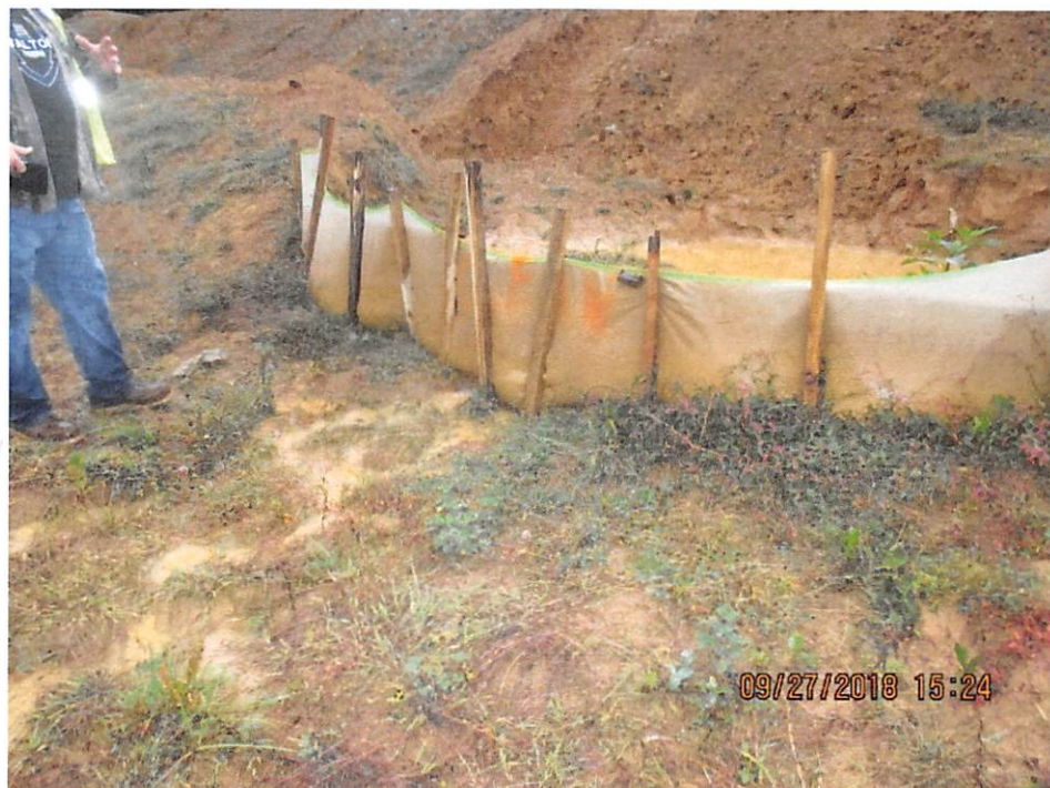
Sediment laden water passing through/under BMP.
