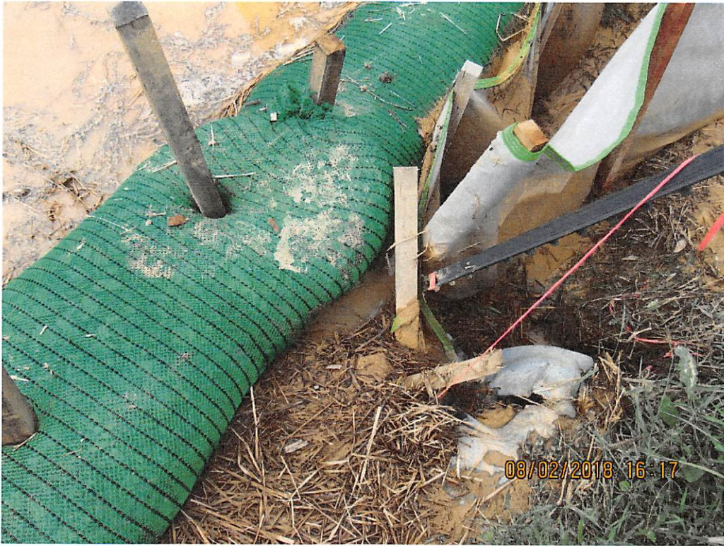
Sediment laden water entering culvert.
