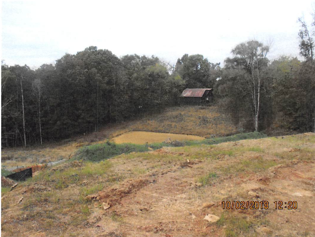
Pond (P-D1) impacted by visible settleable solids.
