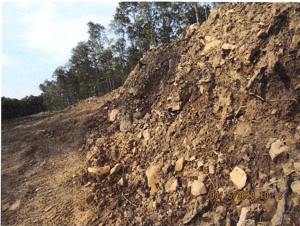
Photo 20: Southern view of waste pile with inadequate stabilization. (Photo taken near Bingham Road station 7450+00)
