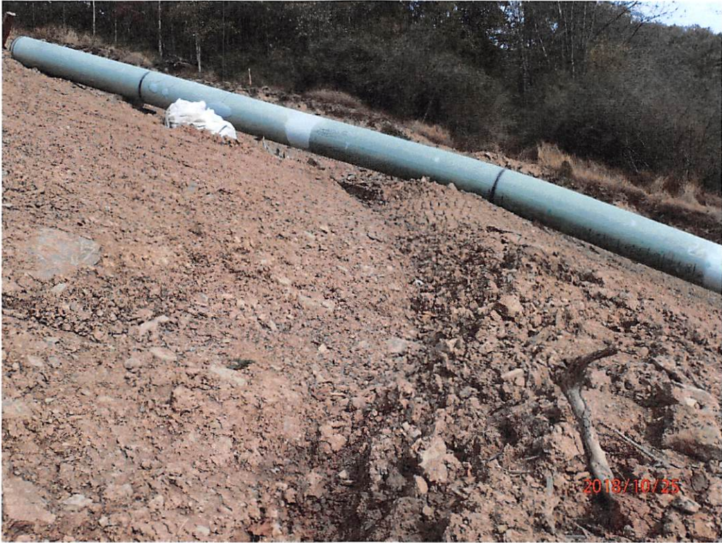
Damaged waterbar directly N of Sams Run.
