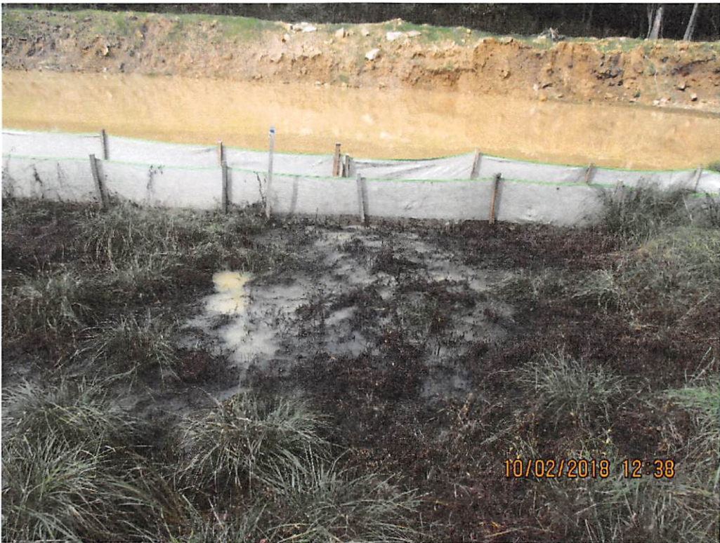
Sediment laden water infiltrating pond P-D2.
