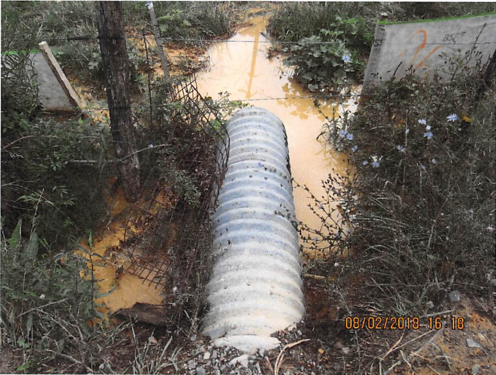
Culvert outlet into wetland area across road from full sump.
