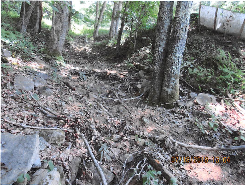
Photo 15: Scour through woods off limits of disturbance upgradient of sediment deposits in Photo 14.
