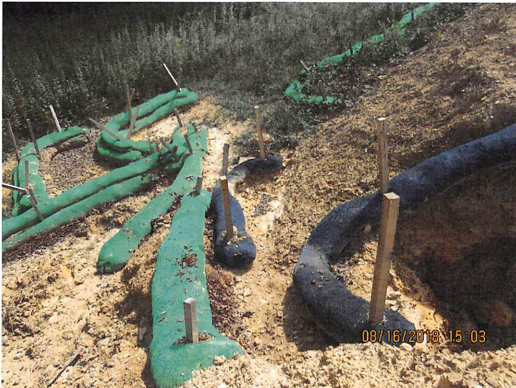
Photo 32: Site of historical water bar terminus control failure- sump installed has reduced failure.
