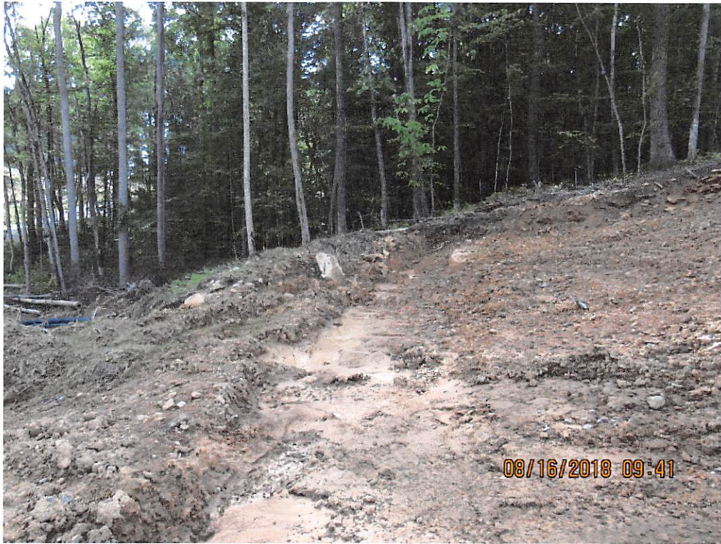
Photo 1: Eastern view of one of several incorrectly sloped water bars off Bingham Road station 7450+00.
