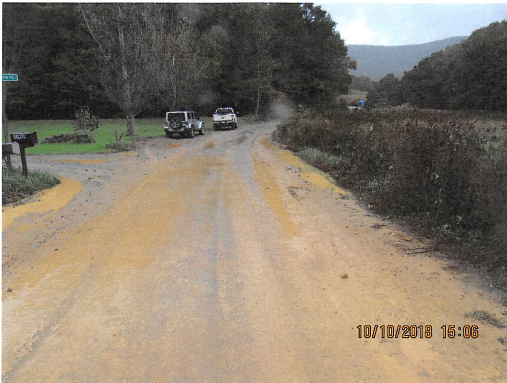
Photo 6: Painter's Run Road station 10270 down gradient of access road crossing.
