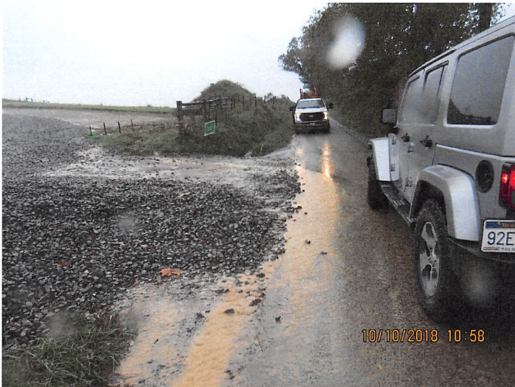
Photo 2: AR 210-sediment laden water leaving site entering county road- up gradient view.
