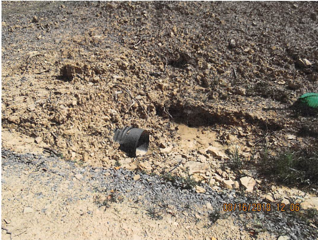
Photo 27: Installed culvert inlet near 7080+00 conveying sediment laden water from water bar terminus in photos 23-25 to SR culvert.
