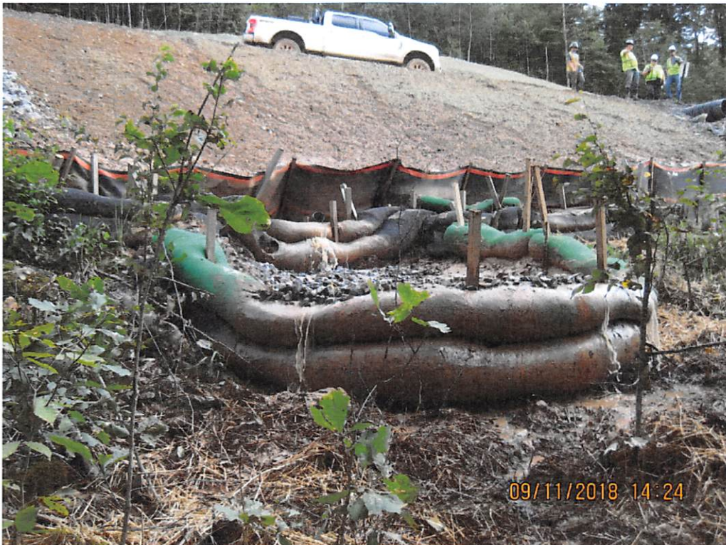
Photo 10: Station 900 (approximately)- upslope view of controls and sediment laden water leaving site.
