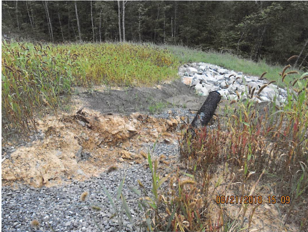
Photo 1: Unfinished underdrain installation.
