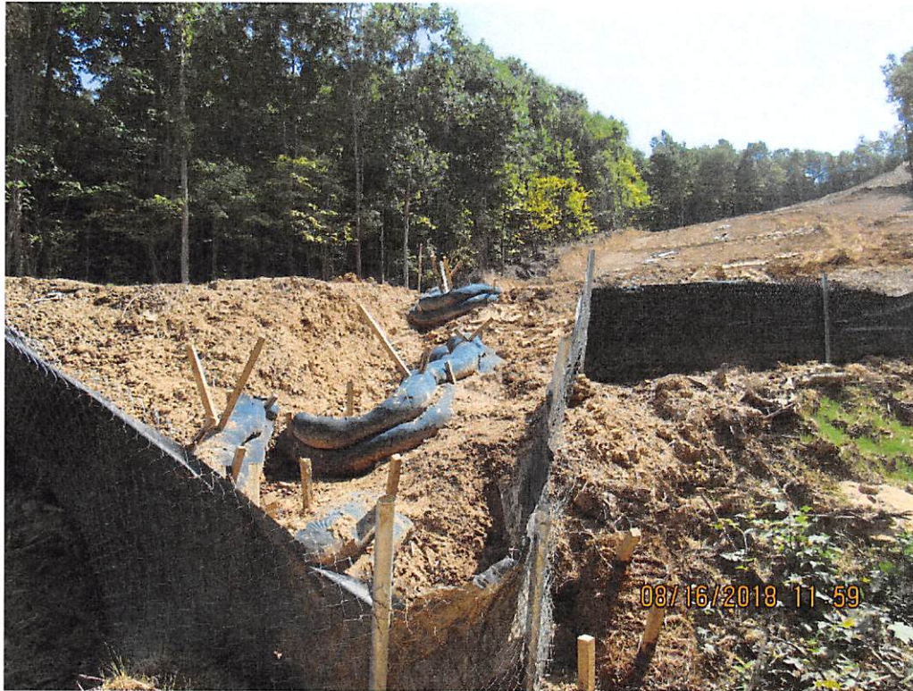
Photo 23: Water bar terminus at station 7084+00 with ROW slope of Photo 21 in background.
