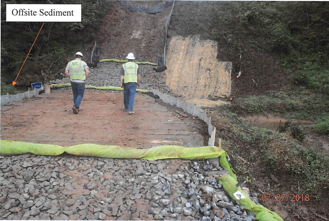
Overview of Grass Run crossing.
