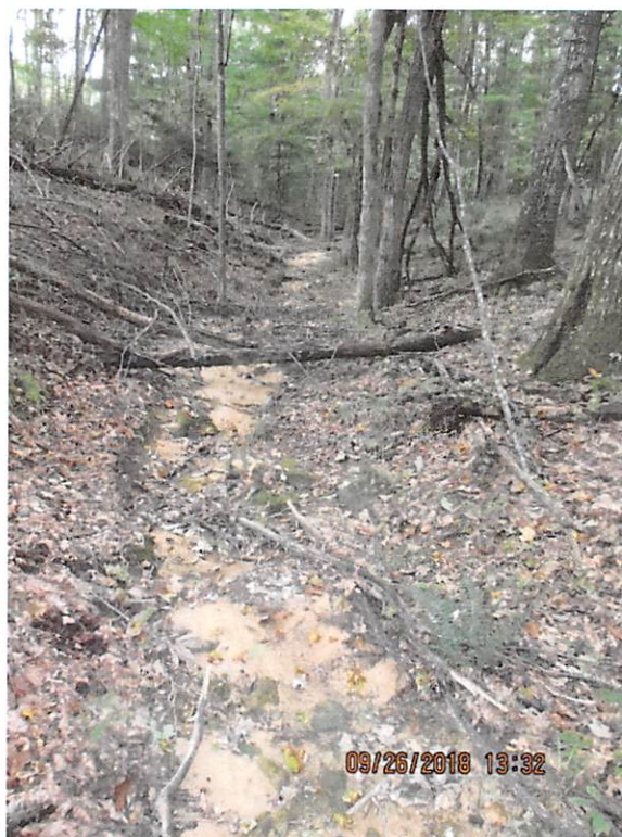
Stream S-H58/TTWV-S-E58 with sediment deposits heading towards Hans creek between Station number 9892+00 through 9899+00.
