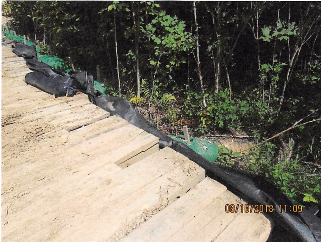
Photo 35: Recommended to add additional controls to timber mat bridge adjacent to wetland at station 7232+00.
