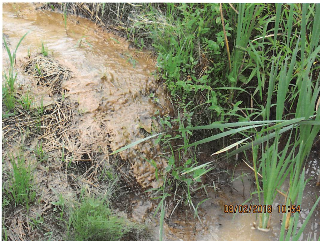
Sediment has been deposited on bank protection product, which is being picked back up prior to entering stream
