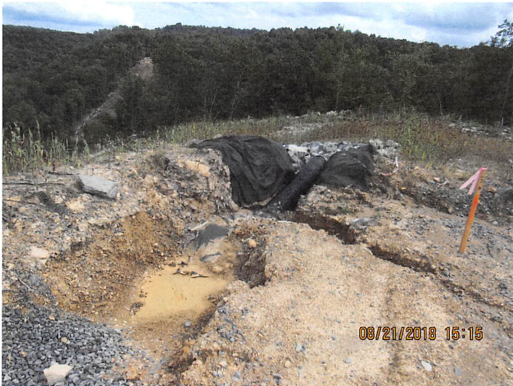
Photo 2: Unfinished underdrain installation.
