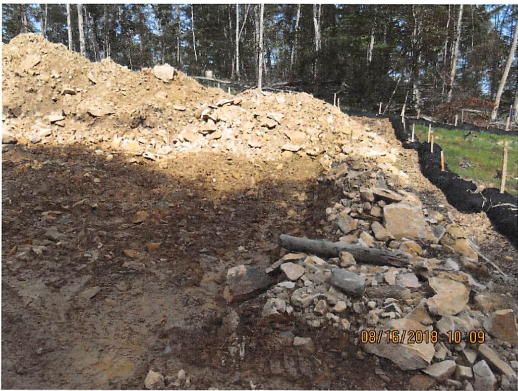
Photo 6: Western view of water bar without outlet near Bingham Road station 7450+00.
