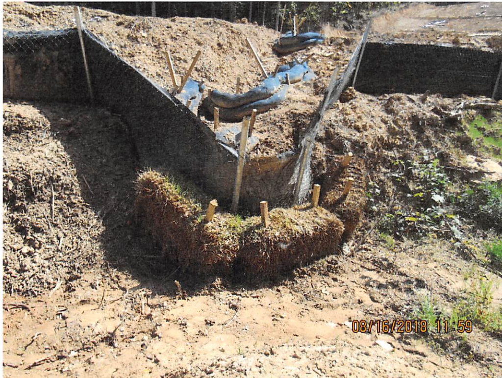
Photo 25: Controls and sediment deposits in road side ditch at water bar terminus at station 7084+00.
