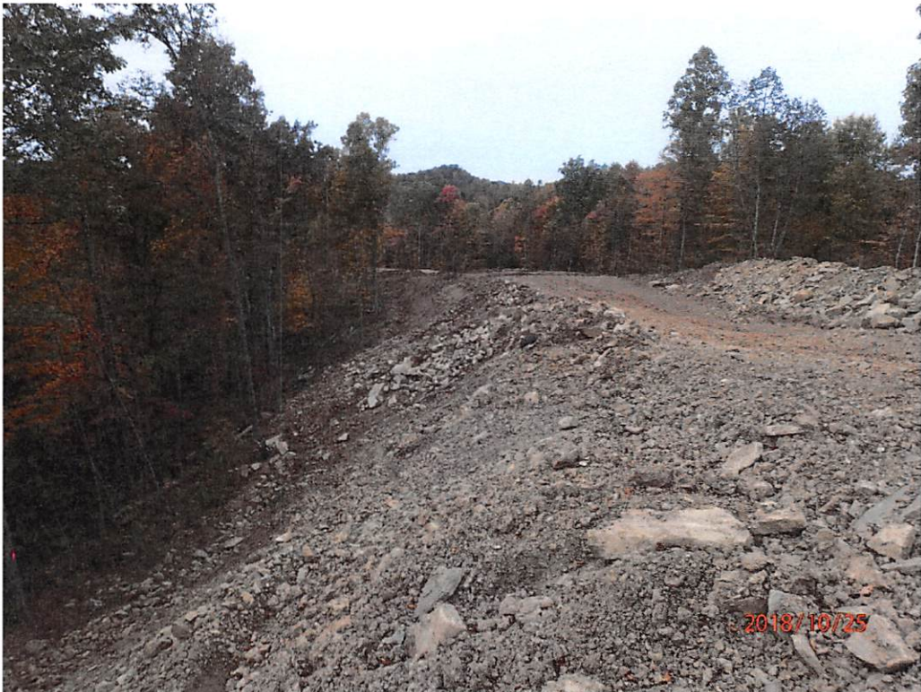
Slip at station 493 had entered the ditchline from a sideslope allowing sediment to leave the project ROW.
