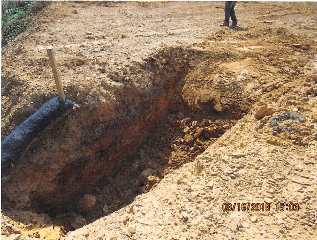
Photo 31: Sumps installed at terminus of water bars near Wahoo Road station 6781+51 which has reduced failure.
