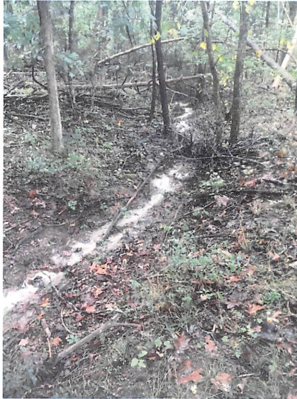
Ephemeral stream near Station #9778+00 being impacted by sediment laden water and flowing downhill and entering roadside ditch at Ellison ridge road.
