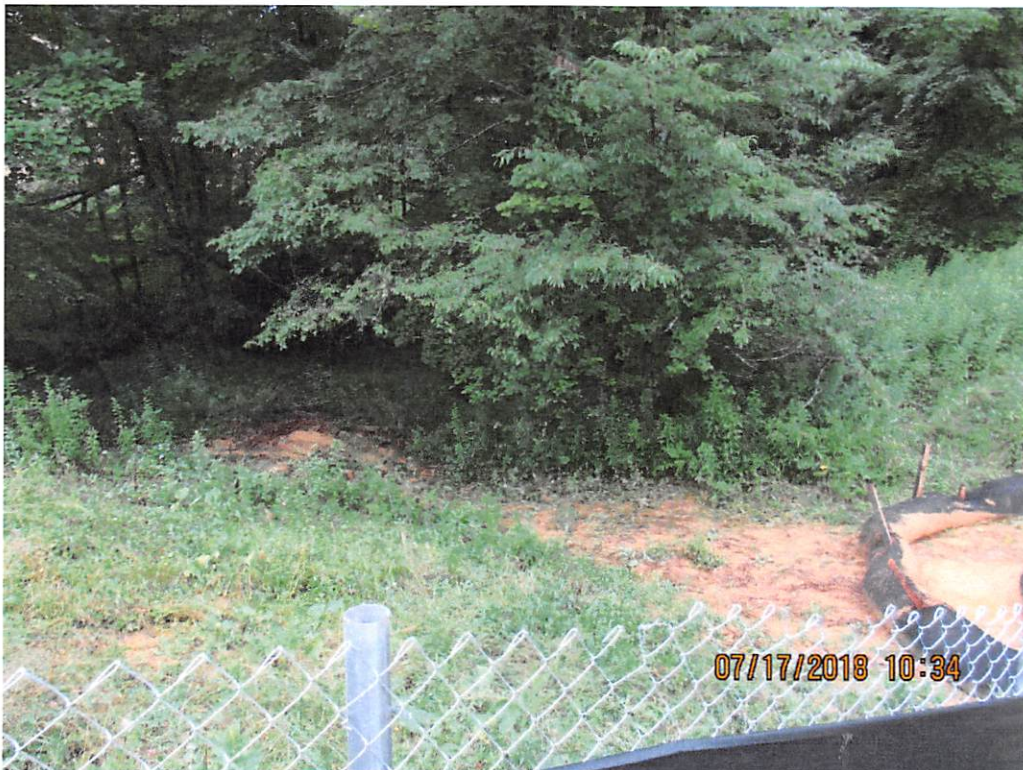
Photo 6: Last compost filter sock in sequence and path sediment laden water created leading to stream.
