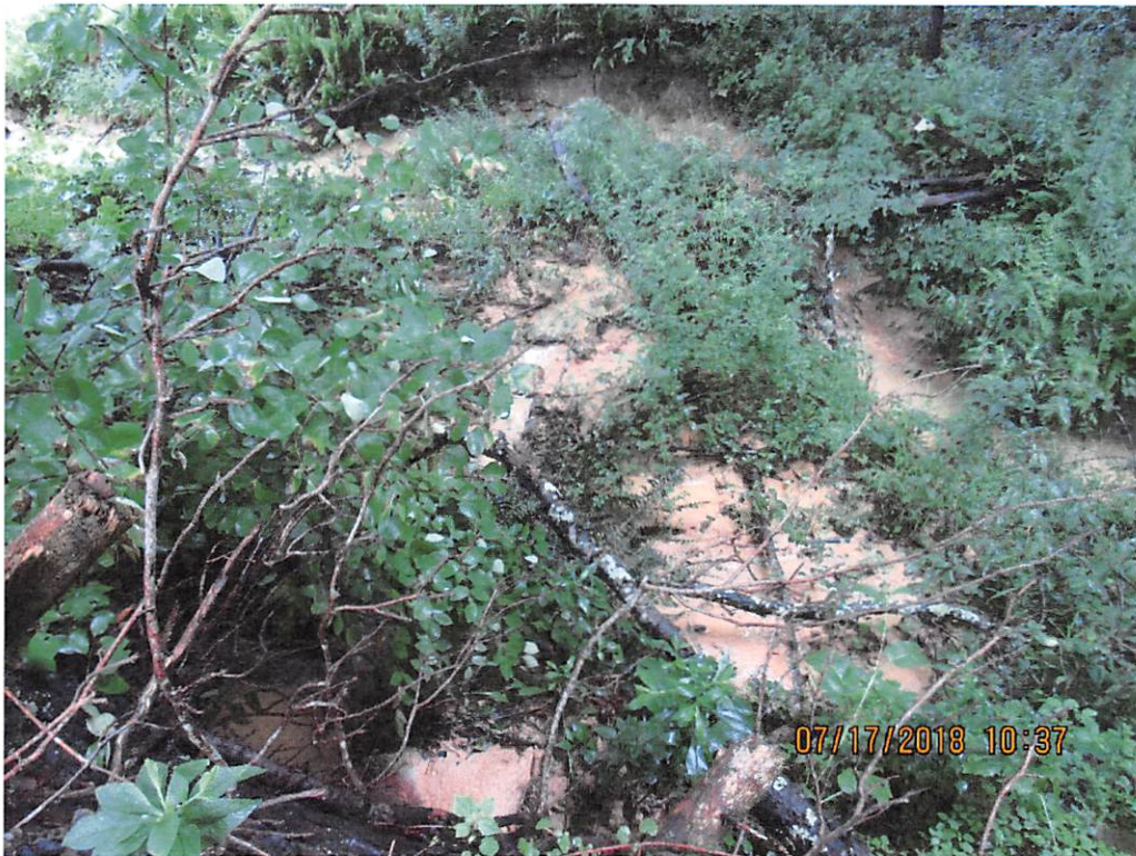
Photo 8: Sediment deposits below temporary tree dam.
