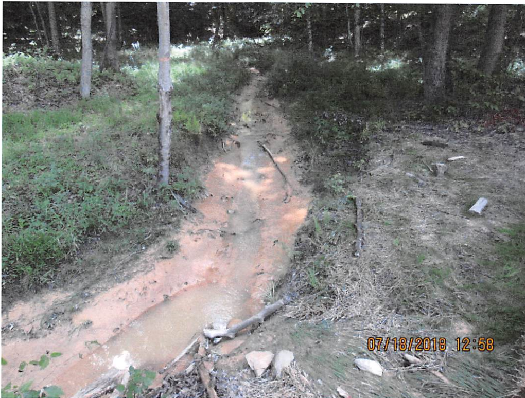
Photo 7: Sediment deposits in UNT of Harmony Creek- upstream of Photo 6. Terminus of control failure in Photos 9 & 10 (vegetation indication under date/time stamp)
