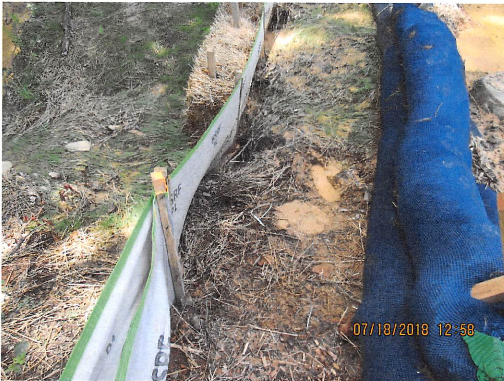
Photo 10: Last control in sequence allowing sediment laden water to leave site.
