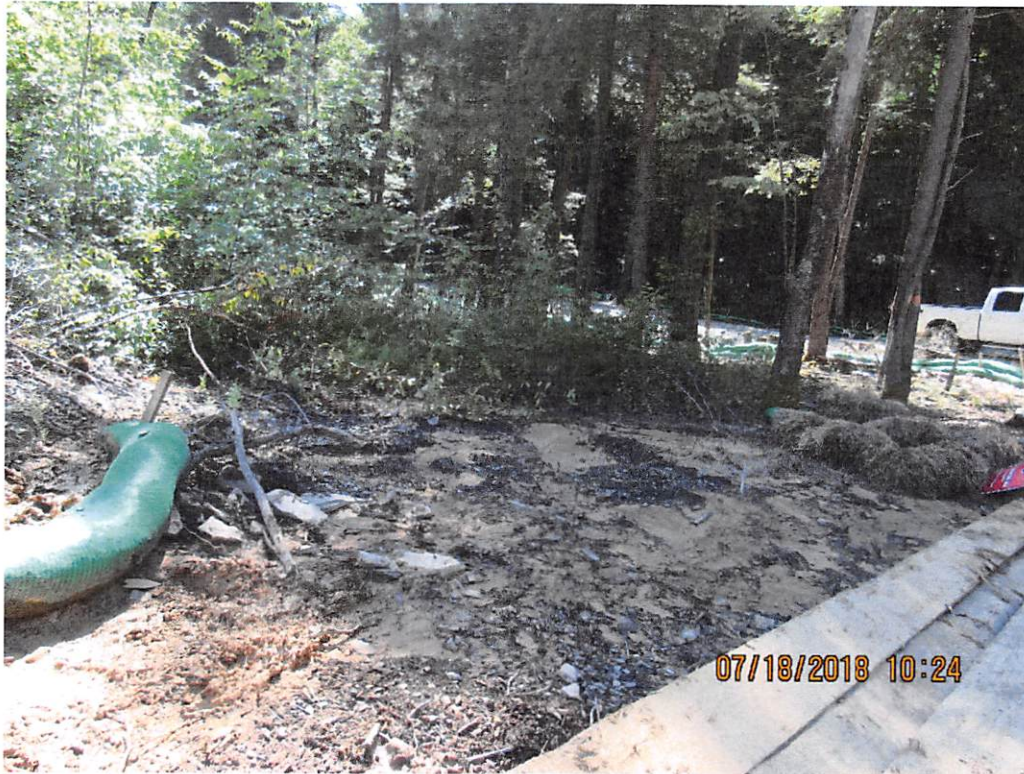
Photo 3: Down gradient of over topped water bar control at station 6898+59.
