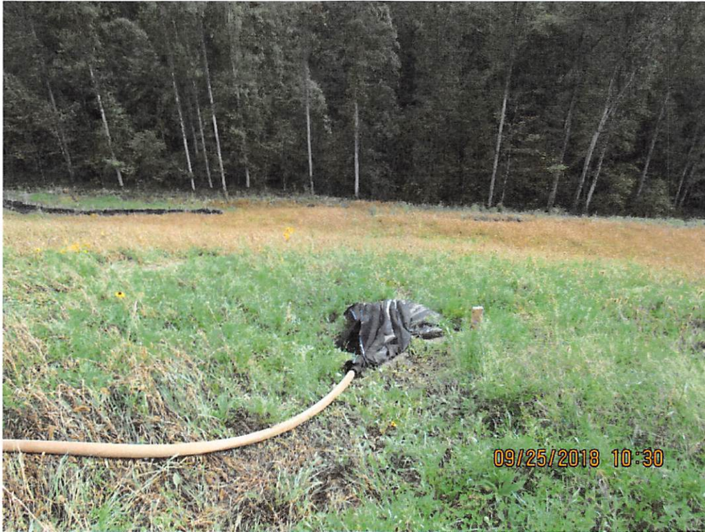
Photo 5: 2 of 3 improperly installed filter fabric bags still in use on north eastern side of site.
