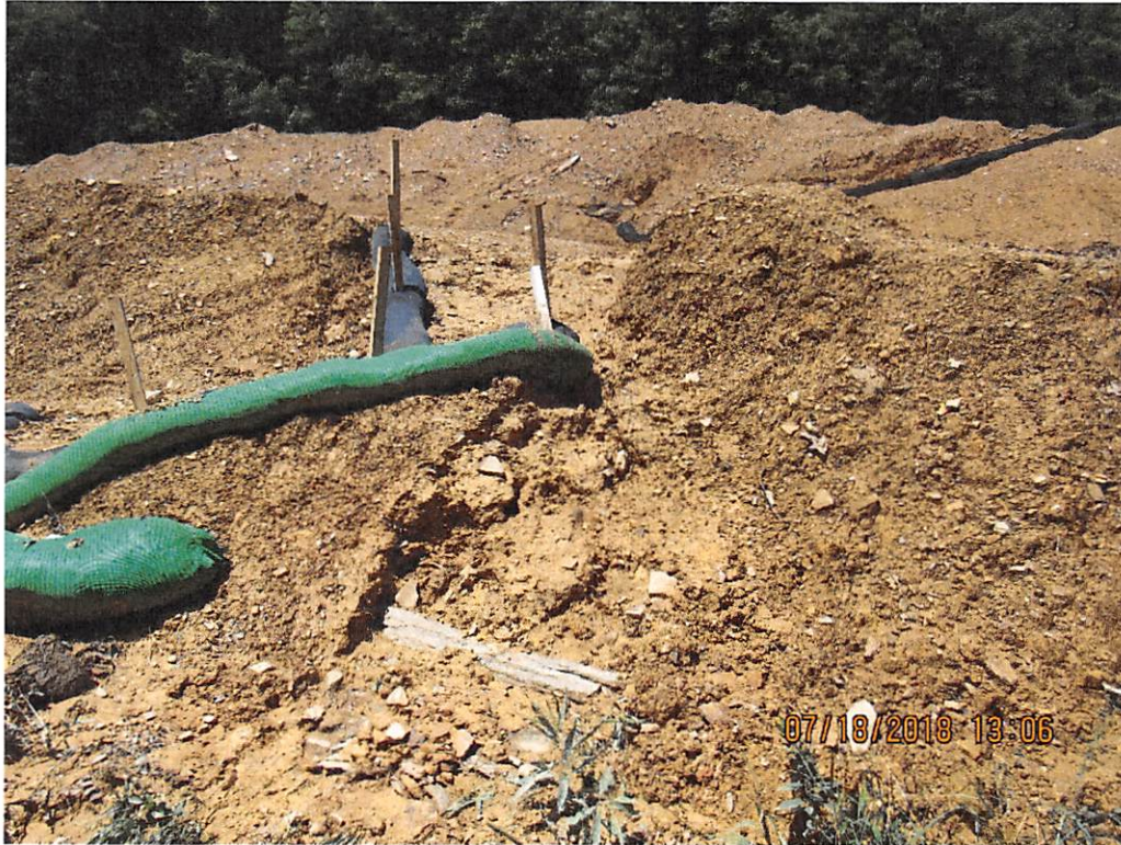
Photo 17: Erosion gullies from failed control at end of water bar near station 6785+50, which allowed sediment laden water to leave site.
