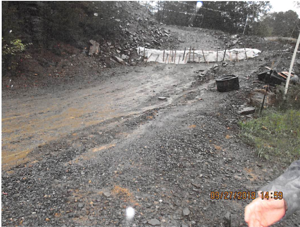
Area where sediment laden water was leaving site and being intercepted by road side ditch along Route 122.
