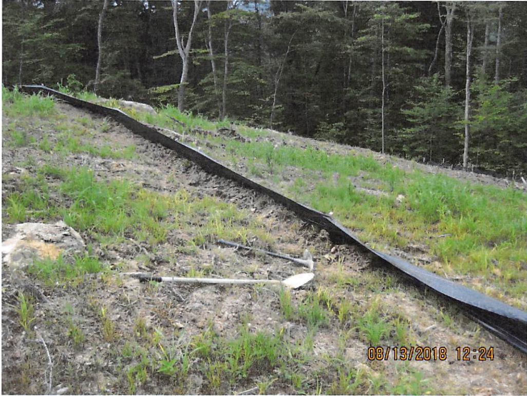
Silt fence being installed on the southern portion of the pad area was not joined or trenched in properly.
