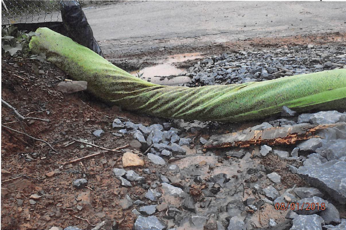
Improperly operated BMP in Right Fork of Big Elk watershed.
