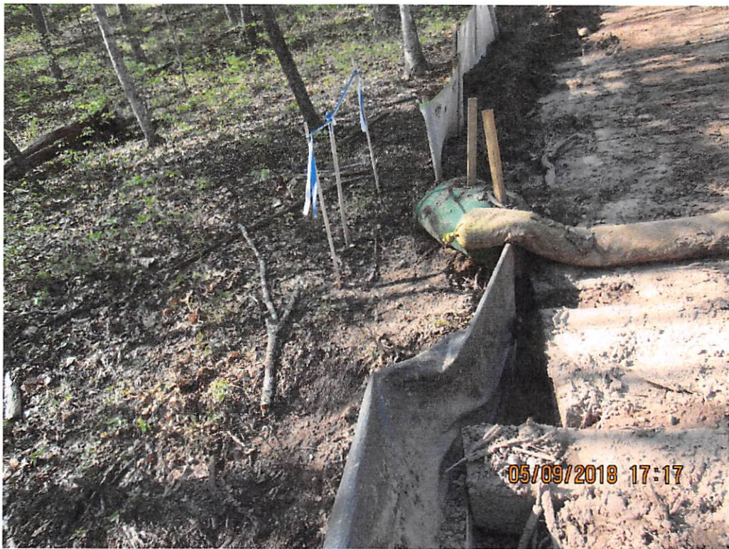
Photo 6: Location of control failure and breach allowing sediment laden water to leave site. Additional control (larger silt sock) added prior to bridge re-build.
