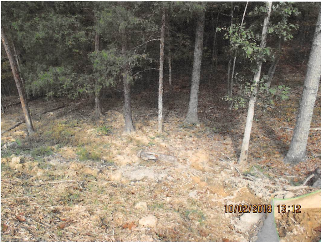
Off-site sediment deposits at Station #9717+52.
